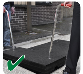
Safe lifting technique with Fibrelite lifting aid.
